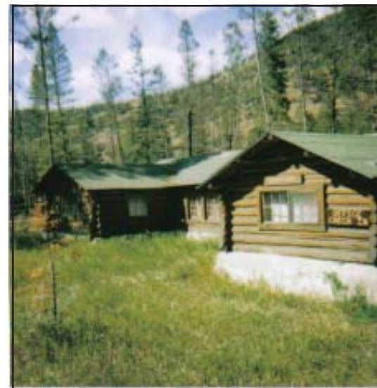
The project to restore the ranger cabin at Camp Buffalo Bill began in the fall of 2003 and was finished one year later with the help of an OA National Service Grant.
