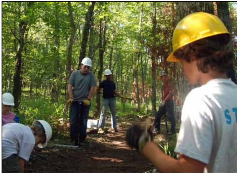
Members of the Ma-Nu-Lodge help build trail.
