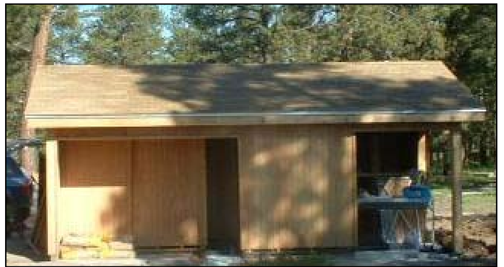
A new bathroom and shower facility was constructed. The facility is completely ADA compliant.
