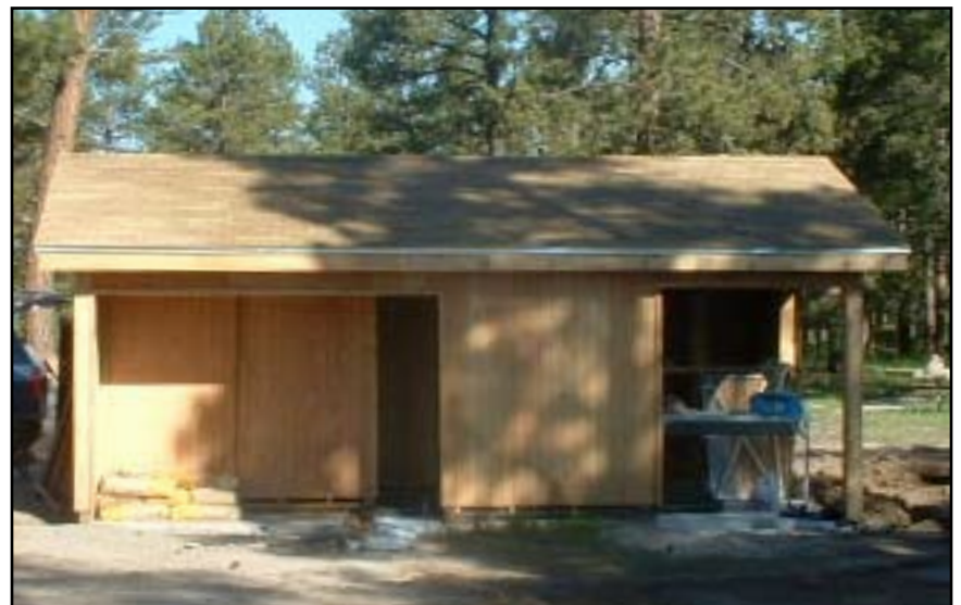
Tahosa Lodge works to renovate a campsite bathroom.
